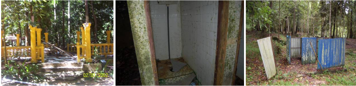
Photo 10: Due to lack in landscape maintenance programmed and system, some of human made landscape elements in Bukit Hijau Recreational Forest cannot be used because of serious damages.
