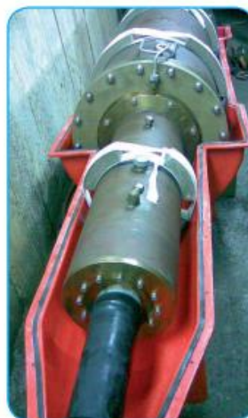
Fig. 4. Transition joint (Prysmian Group 2016).
