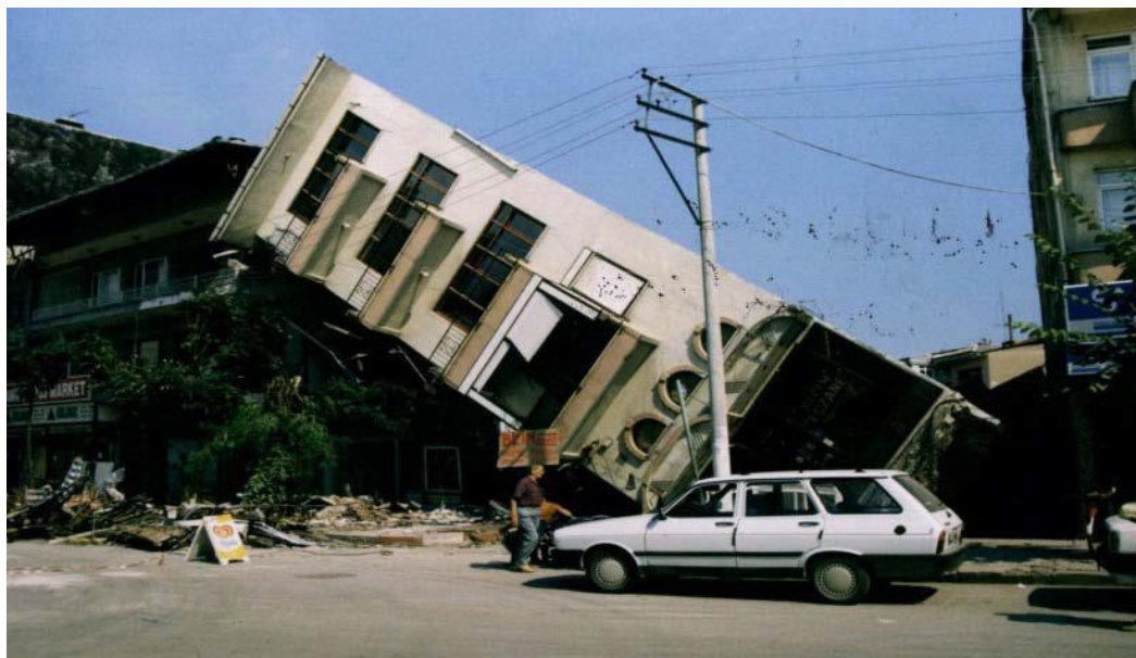
Figure 4. Buildings overturned by liquefaction, during Turkey's 1999 earthquake in Adapazarı Province (Source: http://www.jeofizik.org.tr )
