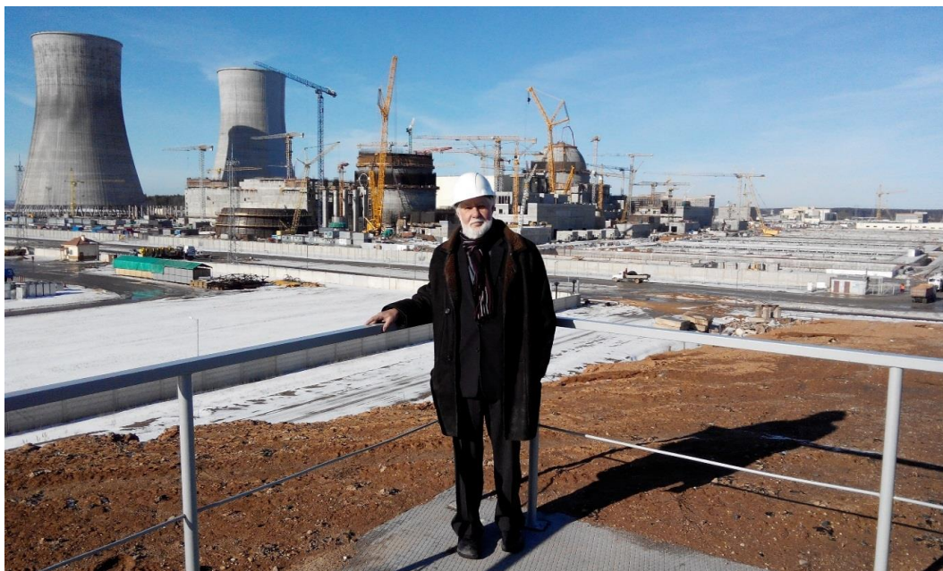
Fig. 5. Panorama of the construction of the Belarusian NPP
