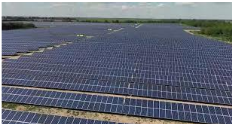
Fig. 6. Solar power plant near the city of Bragin
