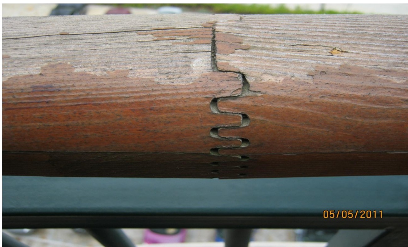
Photo 6. Appearance of coating formed on handle, jointed in length
