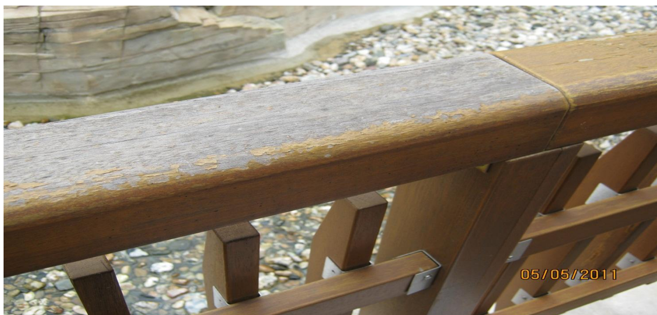
Photo 10. Appearance of coatings formed on parapet handle horizontal surfaces, made of meranti
