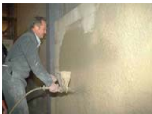
Figure 3. Application by spraying [4]
