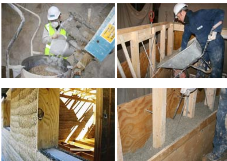
Figure 2. Pouring into boxing [4]
