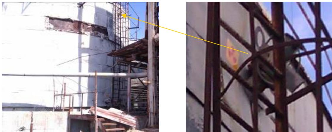
**Figure 15.** Tanks with level switches in the workshop Purified Caustic Soda - the emitters
